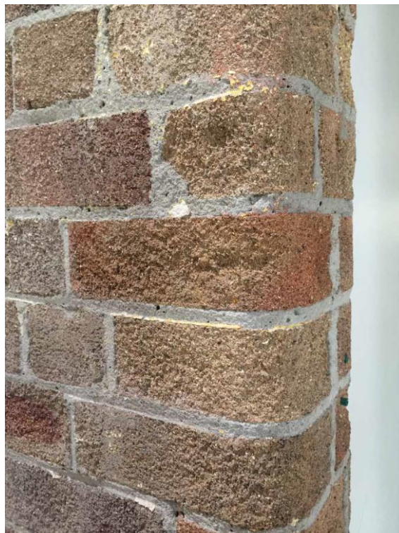
Figure 56 – Brickwork with face reportedly eroded by sandblasting. NBRS Architecture, 2017.
