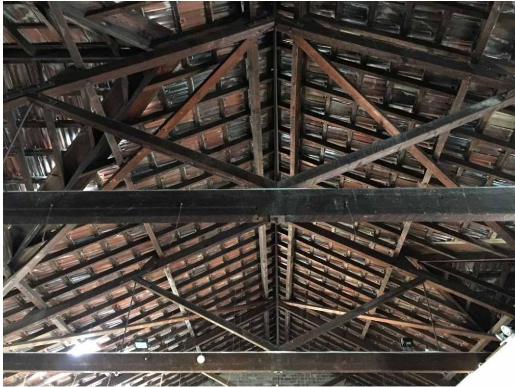
Figure 53 – Timber and steel roof framing over main garage. NBRS Architecture, 2017.
