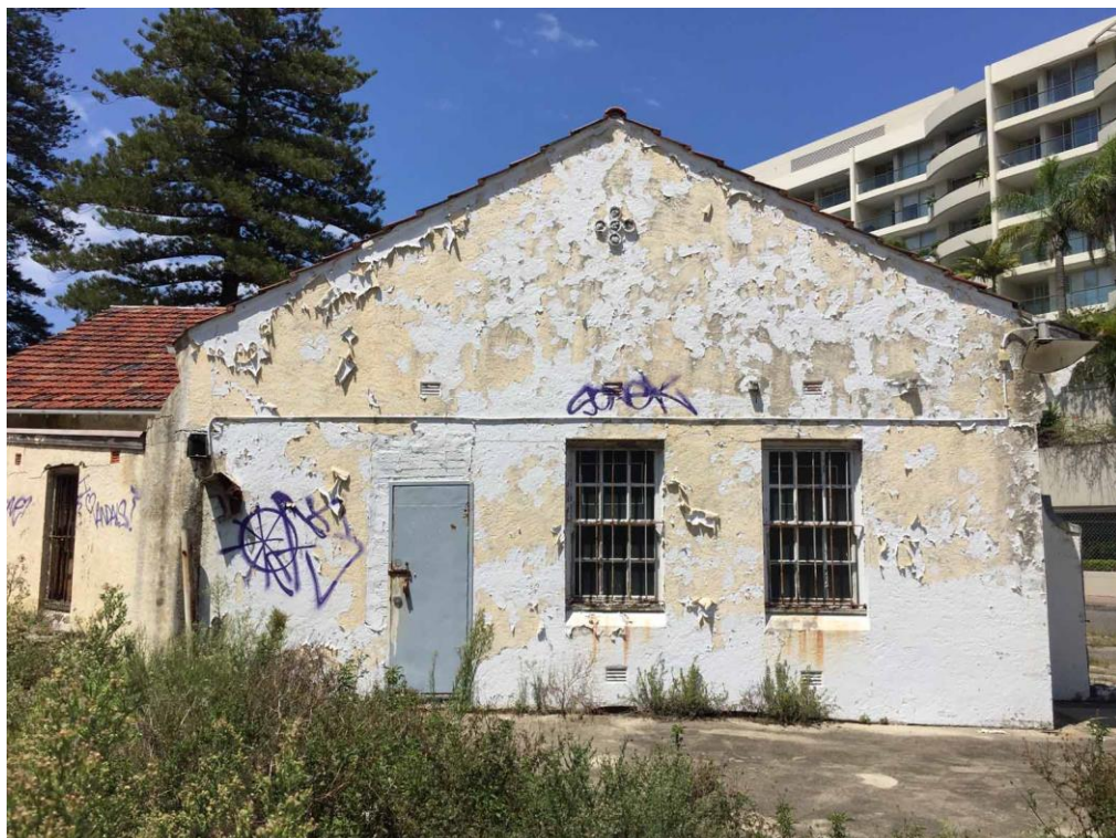
Figure 38 – Rear wall of former garage showing third window with door and bricked up infill. NBRS Architecture, 2017.
