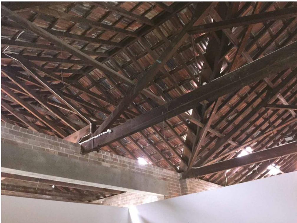
Figure 52 – Roof framing at junction of main and rear garages. NBRS Architecture, 2017.
