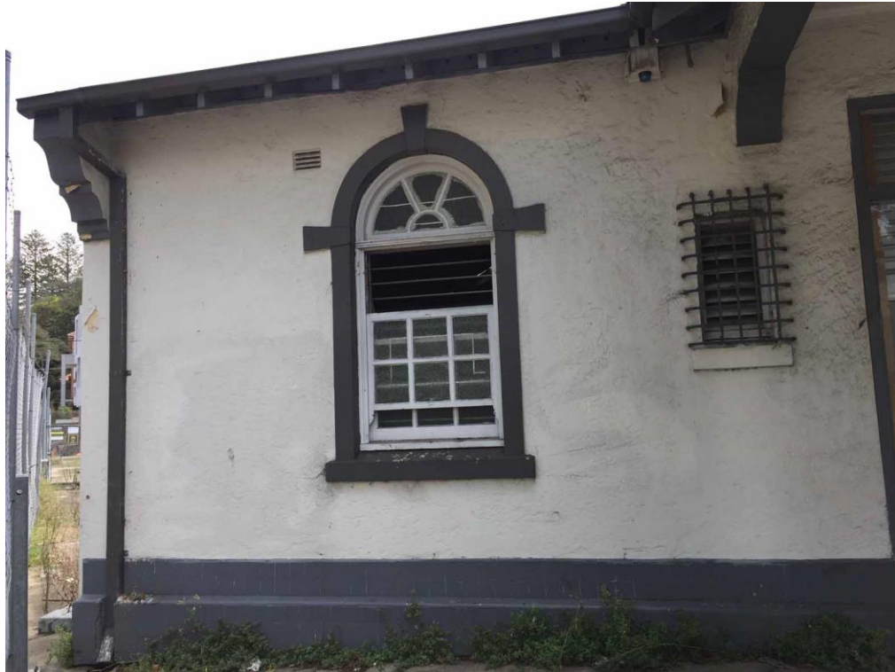
Figure 33 – Detail of front of building showing curved corbels of gable, label moulds to arched window and original wrought iron window grilles. NBRS Architecture, 2017.
