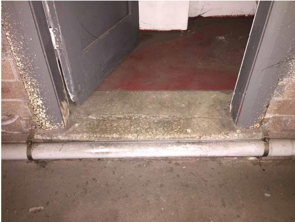
Figure 49 – Damaged terrazzo threshold to toilet. NBRS Architecture, 2017.
