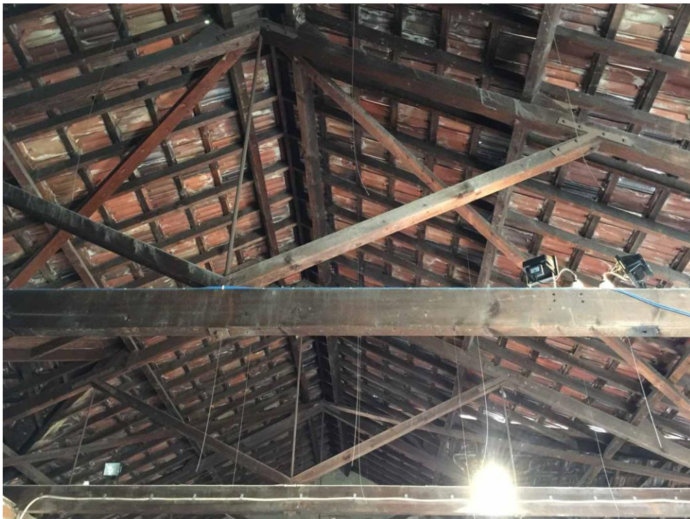
Figure 62 – Roof framing of main garage. NBRS Architecture, 2017.
