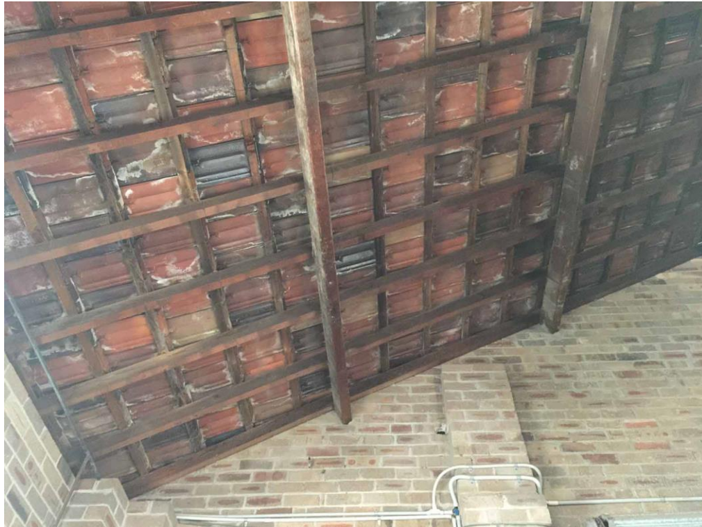
Figure 47 – Underside roof showing salt efflorescence on tiles and leaching onto roof framing. NBRS Architecture, 2017.
